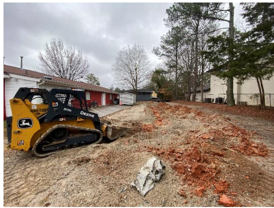
Figure 4. Fixing Parking Area Jan 2024
